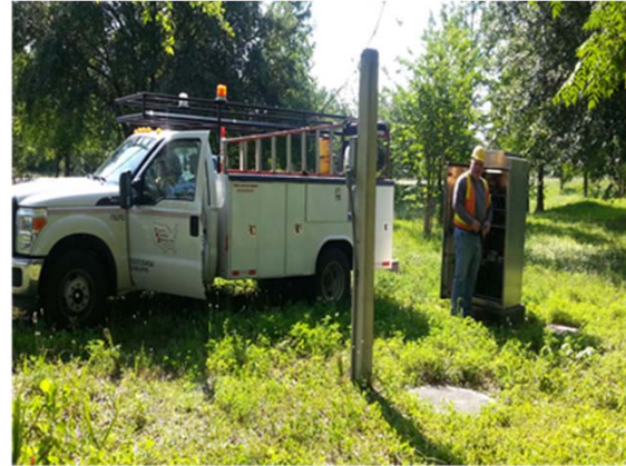
TCD replacing pull boxes
